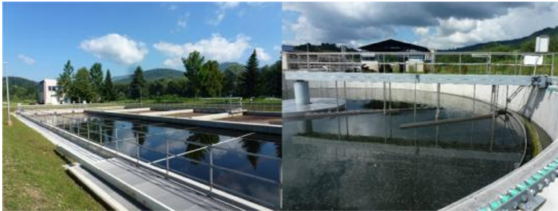
Fig. 1. Rectangular tank in WWTP Dolný Kubín
