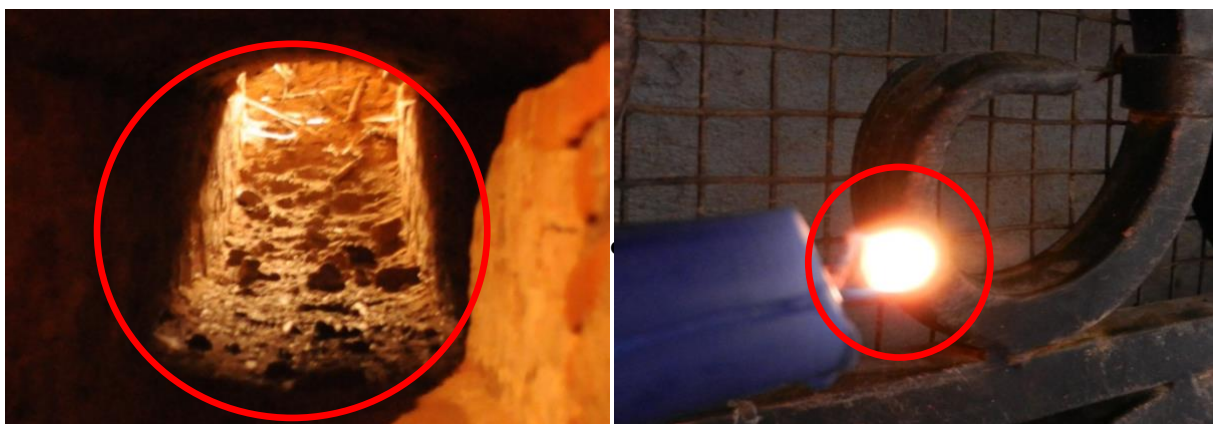
Fig. 2 The ventilation opening of the crypt (left) and a strong flow of the air inside of it (right)
