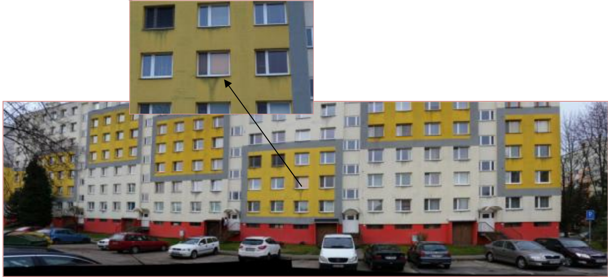
Fig. 1: North Side - contamination by the biological materials (author)
